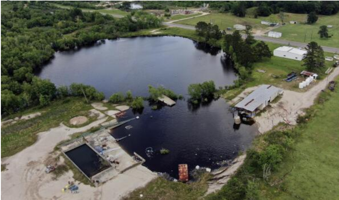
Figure 6.12.5: The Daisetta Sinkhole, 2023
