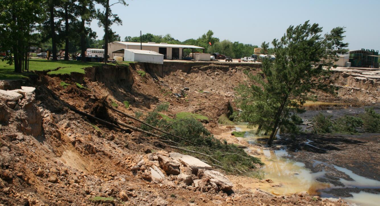
Figure 6.12.4: The Daisetta Sinkhole, 2008
